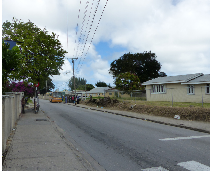
> Street frontage of Civic Campus on Congo Road
